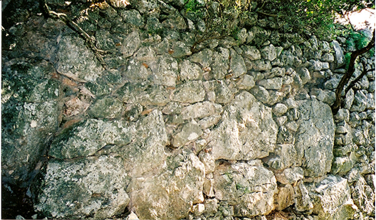
Fig. 35. Castle of Aetos, citadel. View of the W façade. Type 3 masonry.
